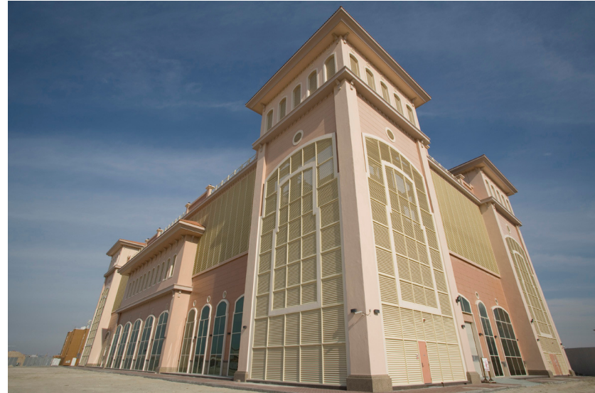
AD 07 – Al Raha Gardens Plant
